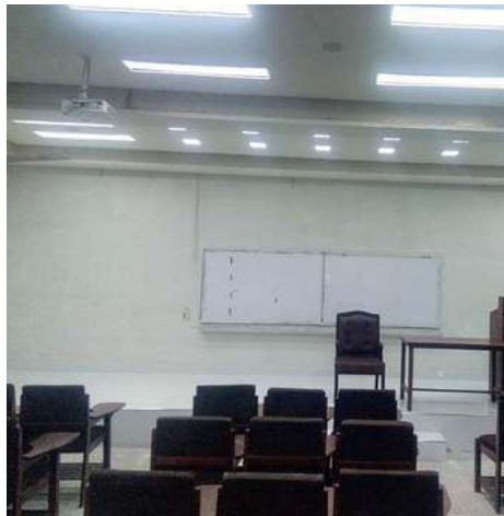
Figure 19: Renovation of Classroom 2
